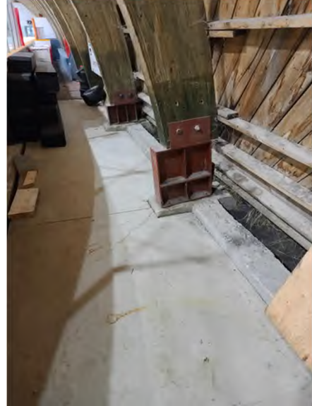
Photo 112 New shoes to the structural frame
