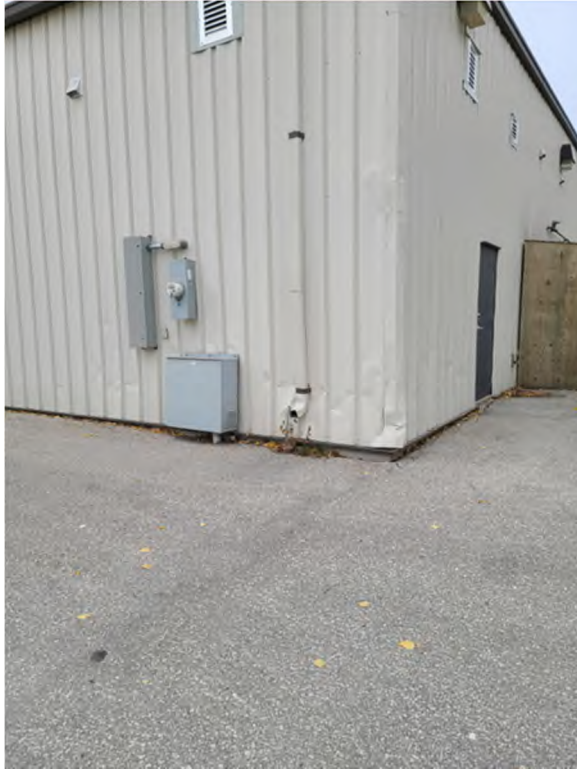
Photo 66 Exterior wall panels
