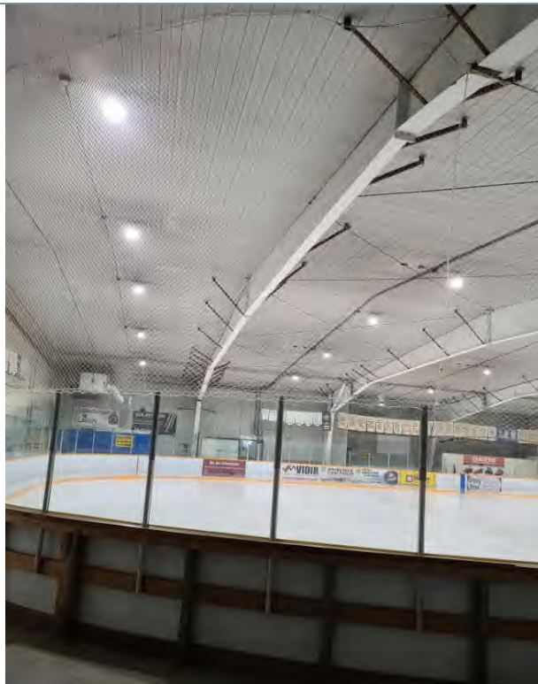
Photo 31 Pre-engineered steel framing in the Arena
