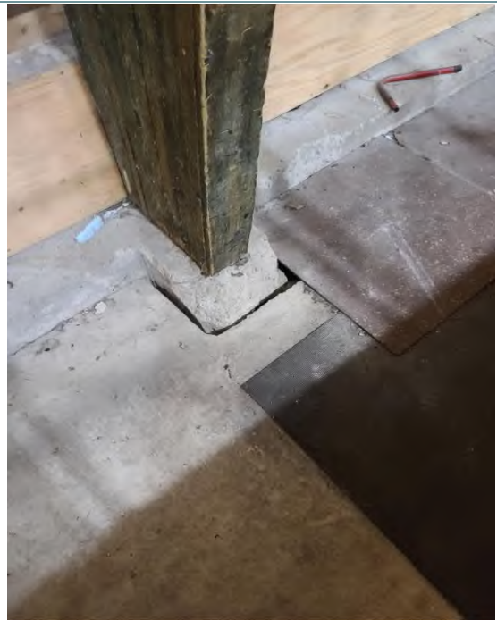
Damages of the concrete grade beam and the pilaster
