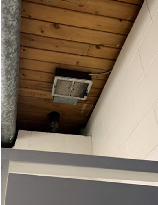
Electric force flow heater in washroom
