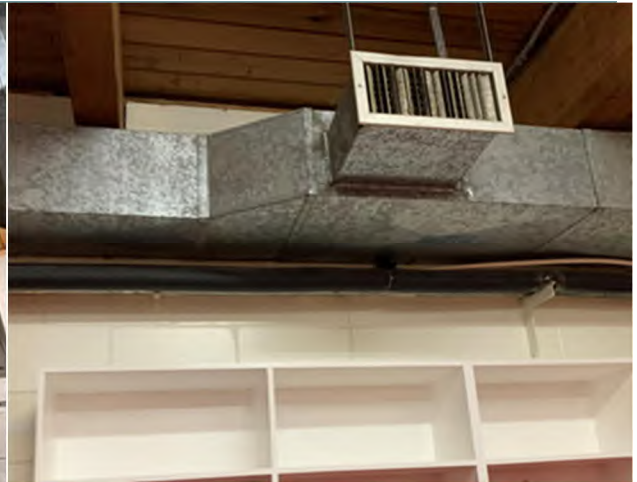
Photo 9 Air handling unit – Electrical Room #2 Photo 10 Age and corrosion in areas of duct work and grilles in dressing room
