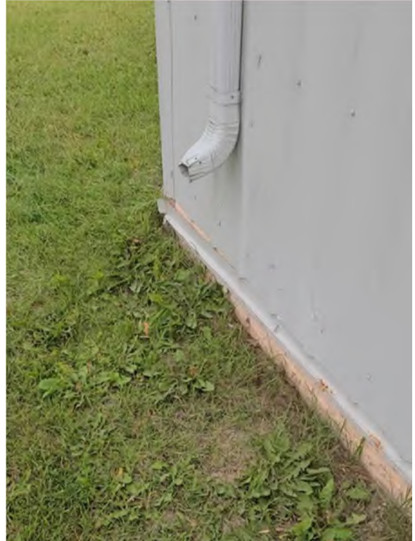
Photo 44 Loose flashing
