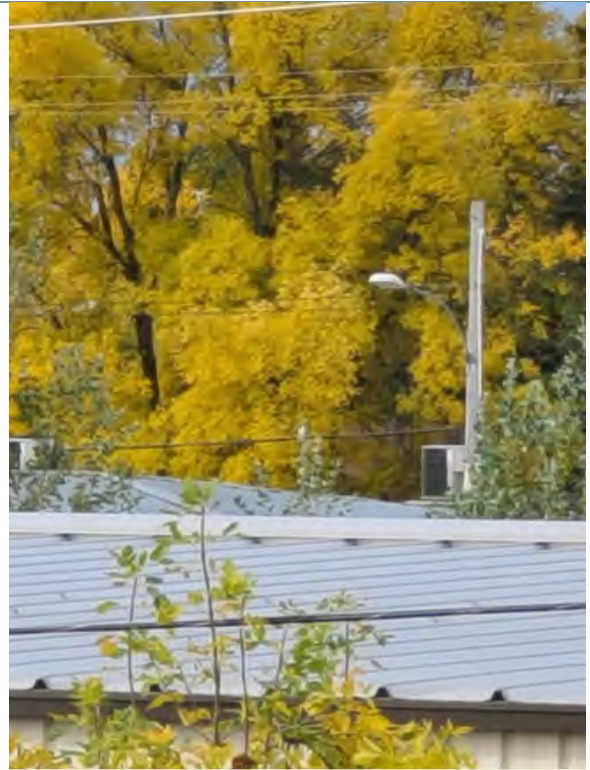
Photo 79 Roof of the Community Center
