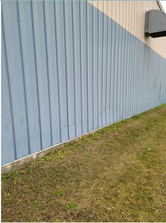
Photo 5 Typical exterior wall panels
