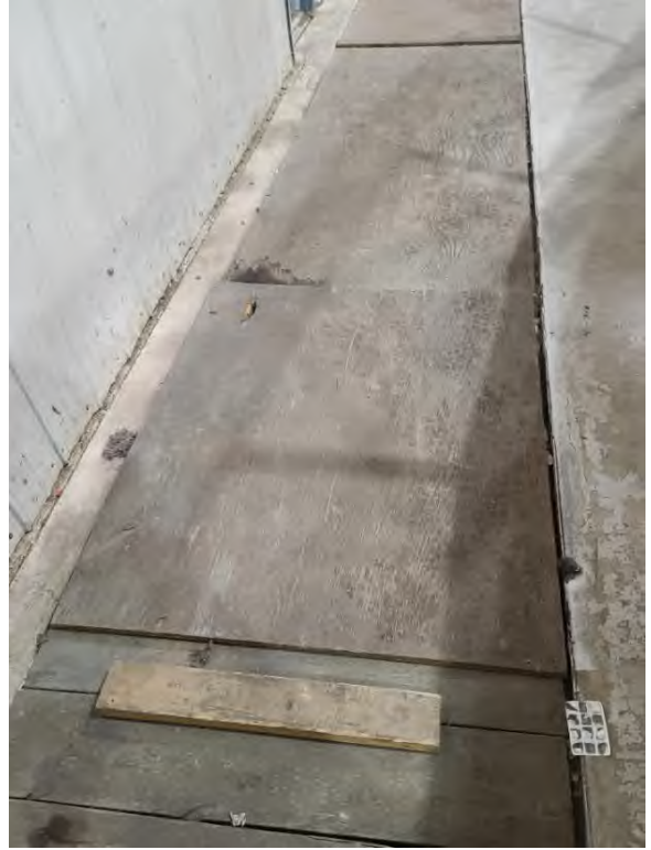
Photo 4 Wood walkway in the arena
