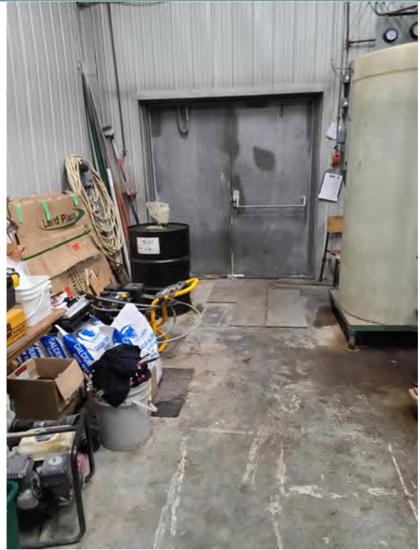
Gap at exterior door threshold in the ice plant
