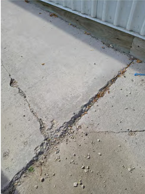
Photo 108 Ramp to the Arena
