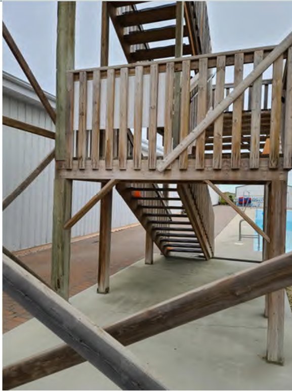
Photo 39 A stair framing to the slider
