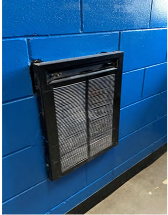
Electric force flow heater in entrance
