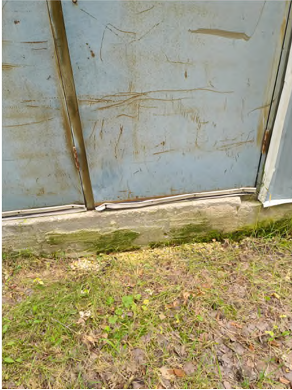
Photo 3 Exterior of an exit door
